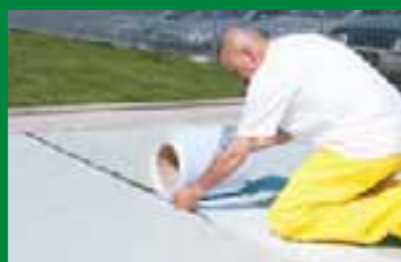
2 FINE TUNED® UNDERLAYMENT ROLLS ARE FIXED TOGETHER
