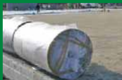
1 THE PREMANUFACTURED MATERIAL IS DELIVERED IN THE BUILDING SITE
