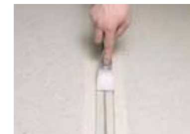
4 Spread the sealing paste with a spatula in both directions in order to make it penetrate uniformly.
