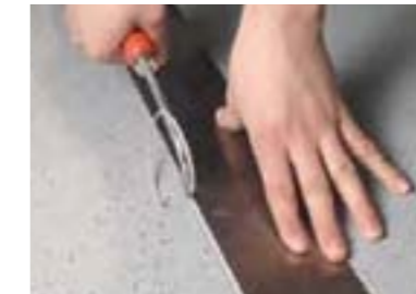
1 Grind joints to a depth of around 1.5 mm according to the thickness of the product
