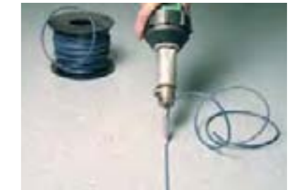
2 Weld with the specific welding tool, setting a temperature of approximately 500°C.
