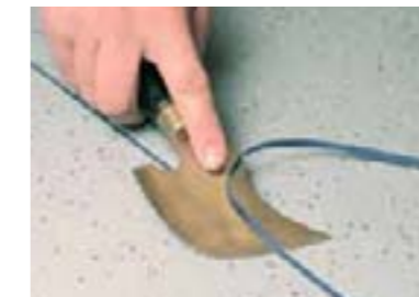
4 Cut flush with the floor using only the 1/4 crescent - shaped knife.
