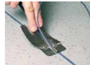
3 Perform the first run using a 1/4 crescent - shaped knife with guide.
